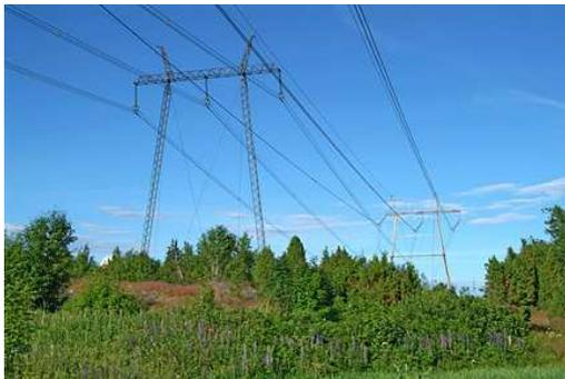
**Figure 2. Transmission line with guyed portal towers**
