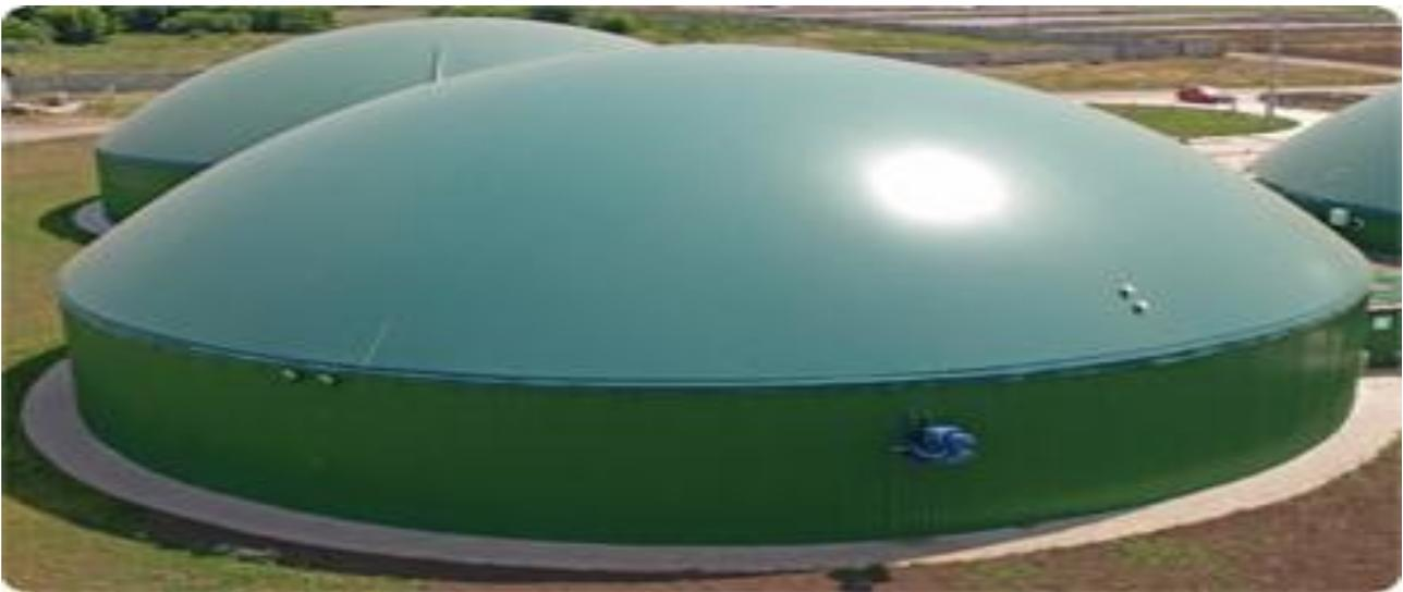
Figure8. Gas holder for biogas [15]
