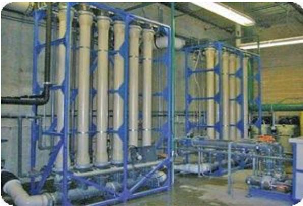
Figure21. Membrane module in operation [23]
