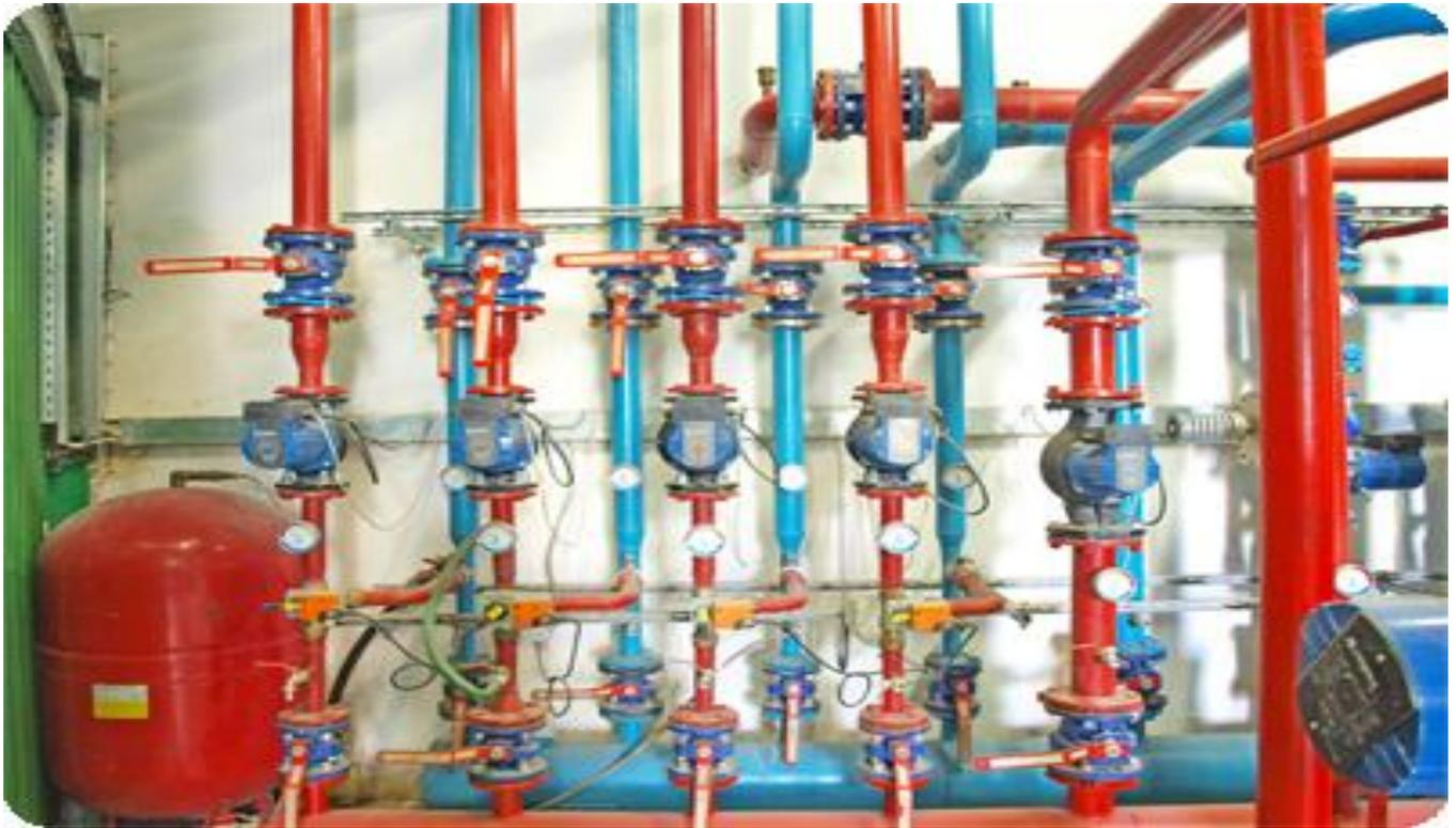
Figure10. Heating unit of biogas plant [16]
