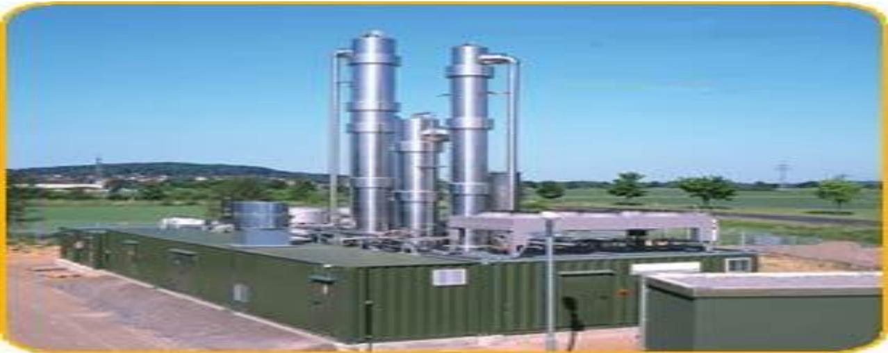
Figure14. Biogas treatment unit 500 m<sup>3</sup>/h capacity [20]
