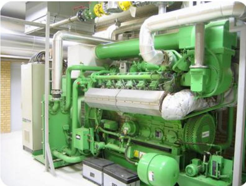
Figure15. Biogas co-generation heat power unit [21]
