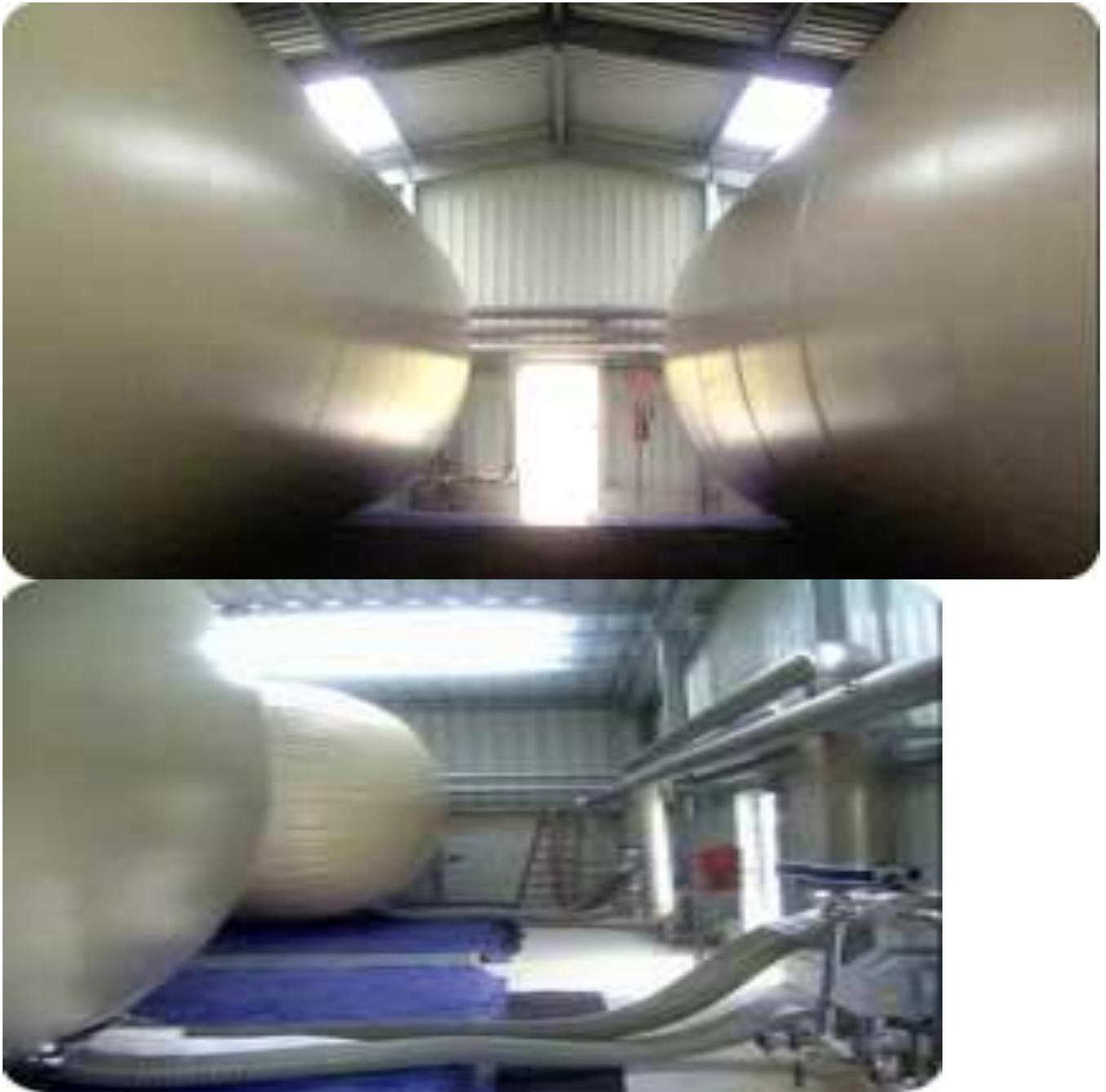
Figure9. Gas holder in special hangar [15]
