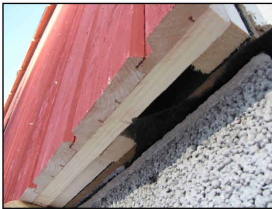
Figure 11. Ventilated Facade
