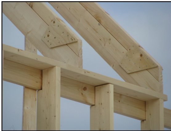
Figure 9. Connections in Roof Frame
