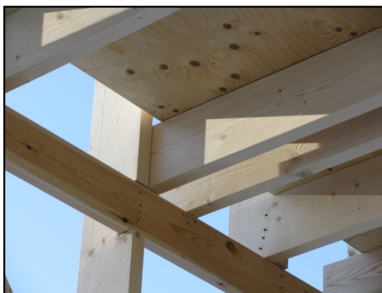
Figure 7. First Secondary Beams
