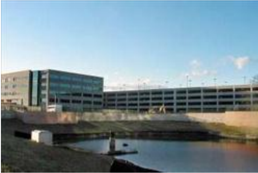
Figure 2.9 The Redbrook Financial Center parking structure, Maryland, USA (VStructural, LLC., 2010)
