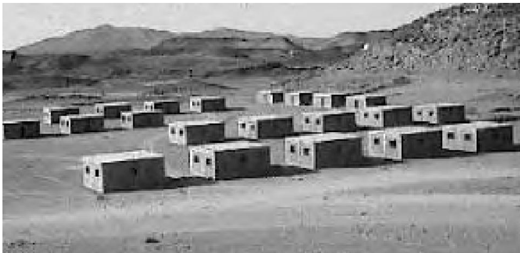
Figure 2: Housing units after Dhamar earthquake 1982 - Source: Sultan Barakat
