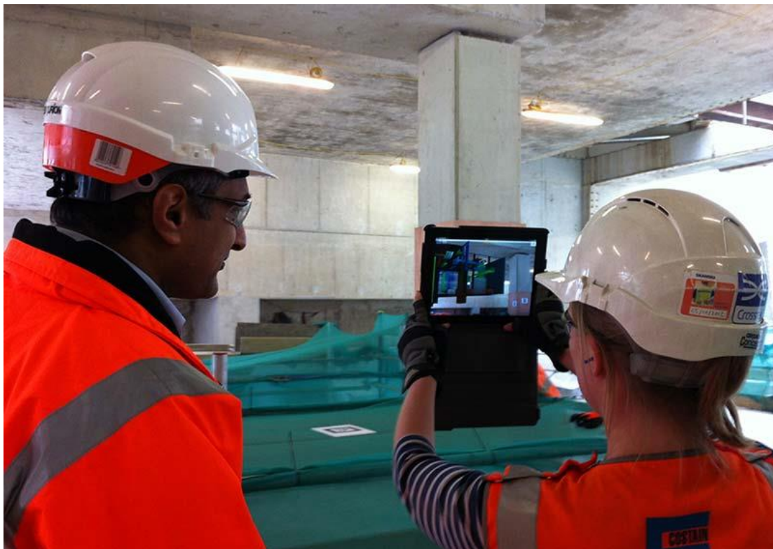
Figure 32 Using an Augmented Reality tool in construction operation. Source: (The Institution of Civil Engineers, 2019).
