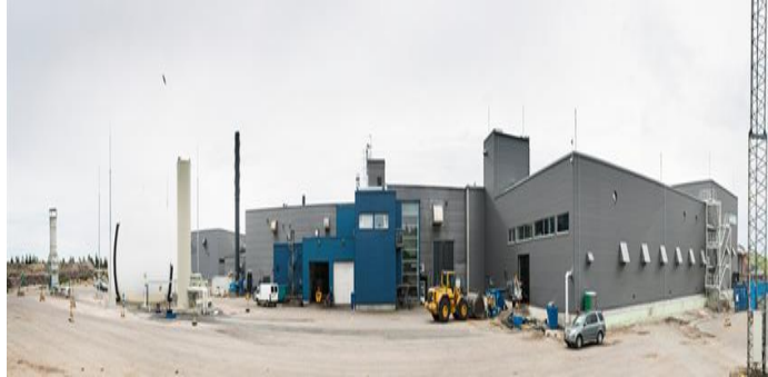
Figure 8. HSY building for waste management, Espoo, Finland
