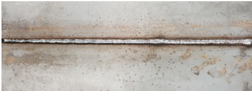
Figure 20 Quality of Second Weld Run
