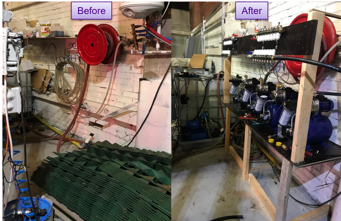
PICTURE 3. Pumps and valve shelf installation (Author 2019)
