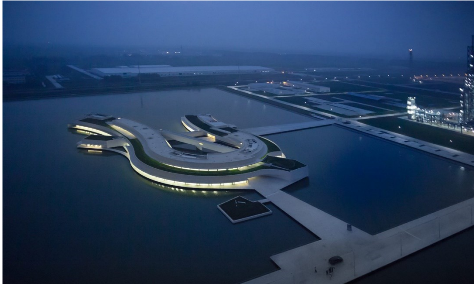
Figure 32. The Building on the Water, Huai'an City (retrieved from https://www.carlos-castanheira.pt/project/the-building-on-the-water/# )
