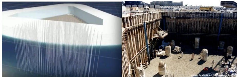
Figure 23. Piles model and Figure 24. Basement excavation work (retrieved from CTBUH)
