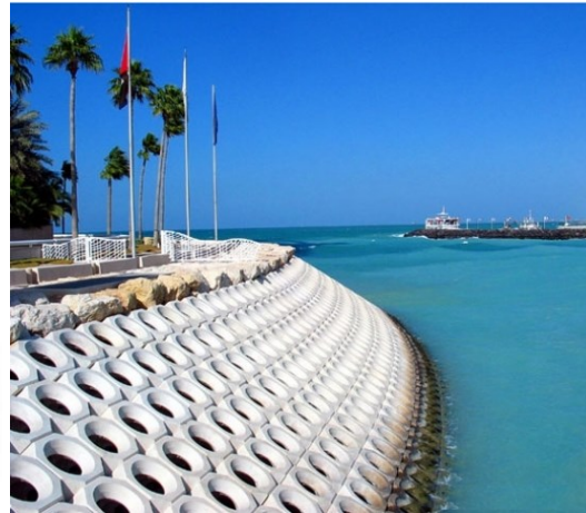
Figure 25. Cubic concrete armour and Figure 26 Shed armouring at Burj al Arab Hotel (retrieved from https://www.xbloc.com/sites/default/files/domain-671/documents/xbloc-2008-design-of-concrete-armour-layers-muttray-et-al-671-14585724381469179232.pdf )
