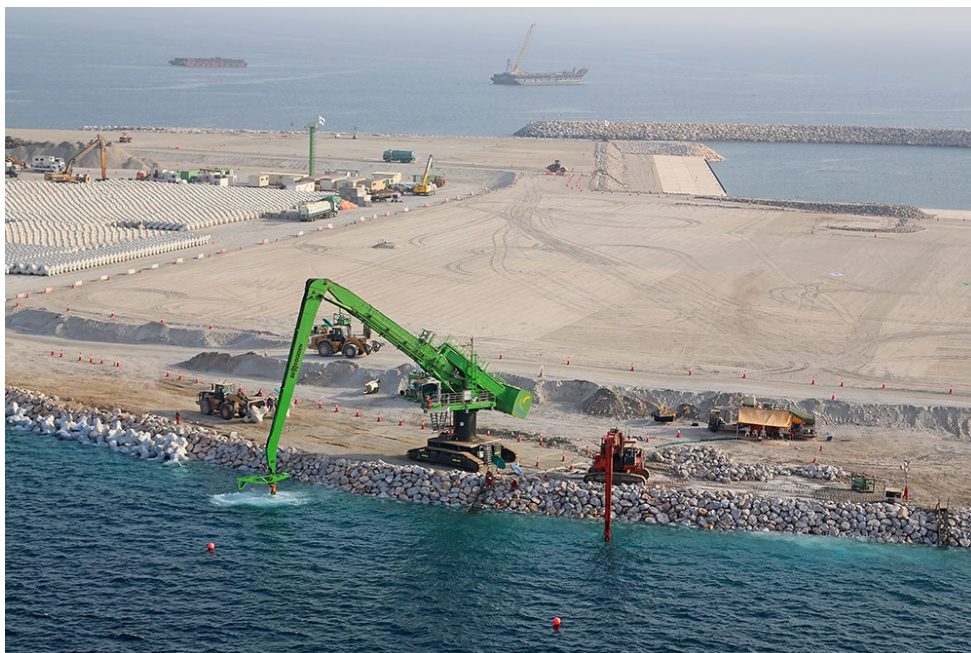
Figure 2. Construction site of the artificial island (retrieved from https://www2.deme-group.com/references/sarb-artificial-islands )
