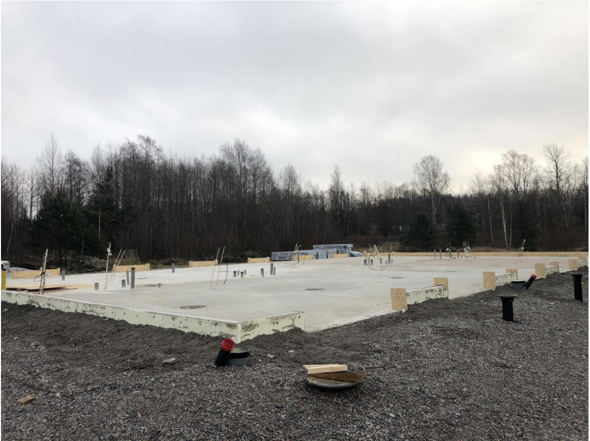
Figure 31. Construction site (November 2020)
