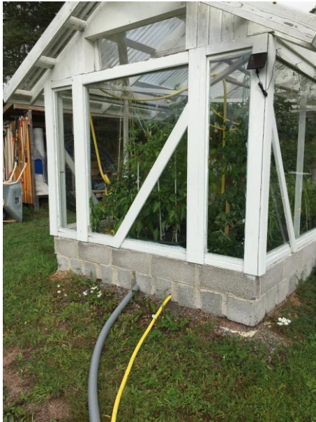
PICTURE 11. Glasshouse. Grey (insulated) pipe for inlet hot water and yellow (non-insulated) for outlet cold water. (Author 2020)
