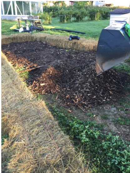
PICTURE 1. Initiating the process. First layer of woodchips applied, and edges delineated with haybales for moisture and heat conservation. (Author 2020)
