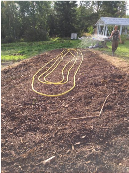
PICTURE 5. Assembled heat collector hoses and watering of feedstock (Author 2020)
