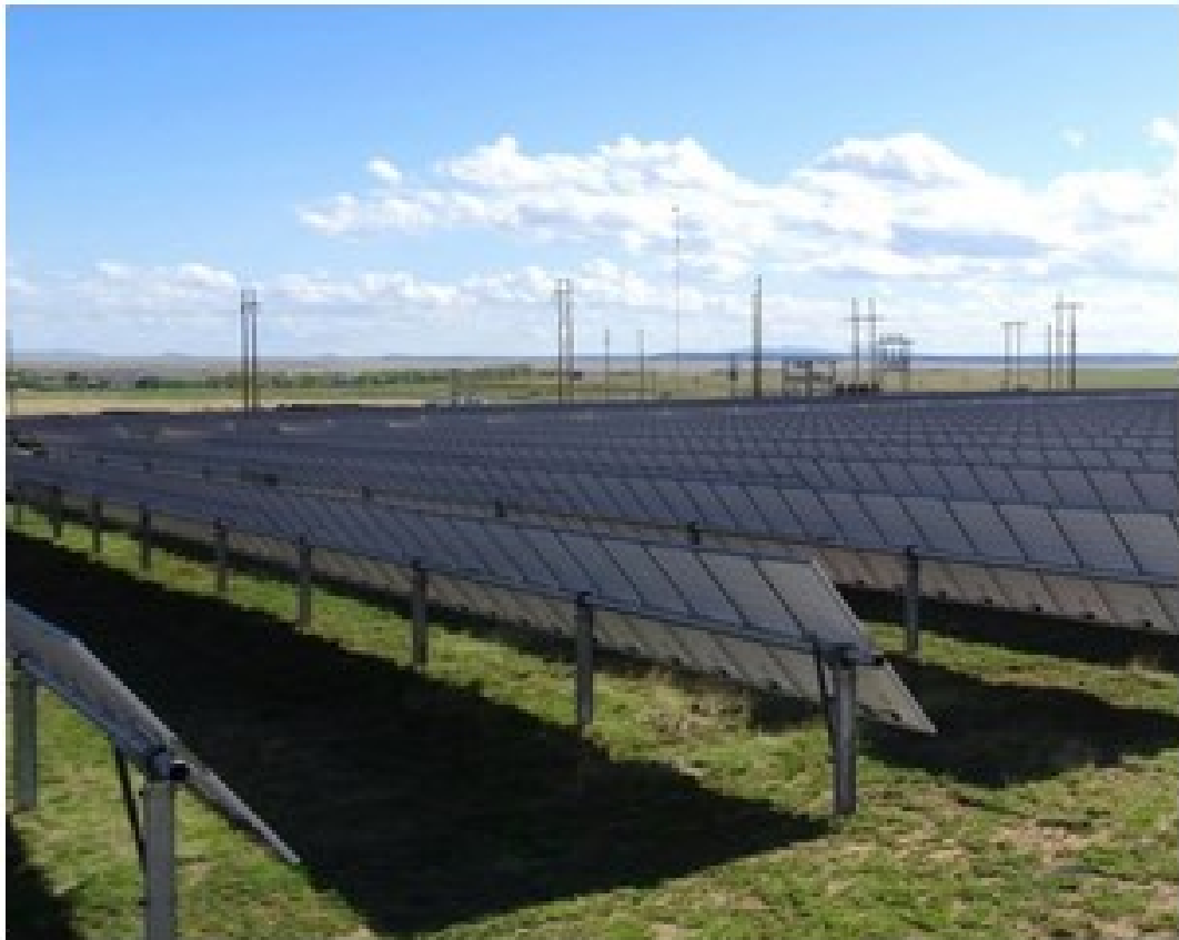
Picture 8 A solar farm with single axis trackers. (Bebon, 2016.)
