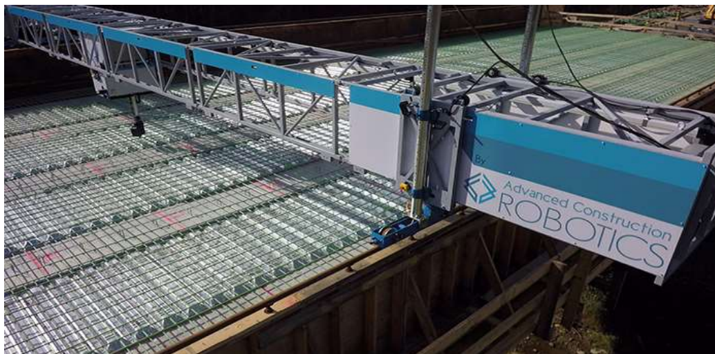
Figure 31: Expanded TyBot arm on Deck's Width 33
