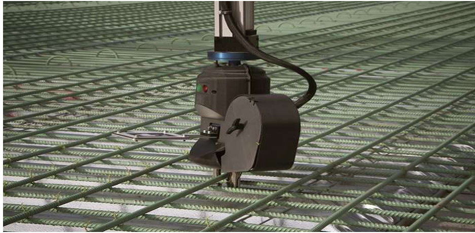
Figure 32: Tying rebar by TyBot 34
