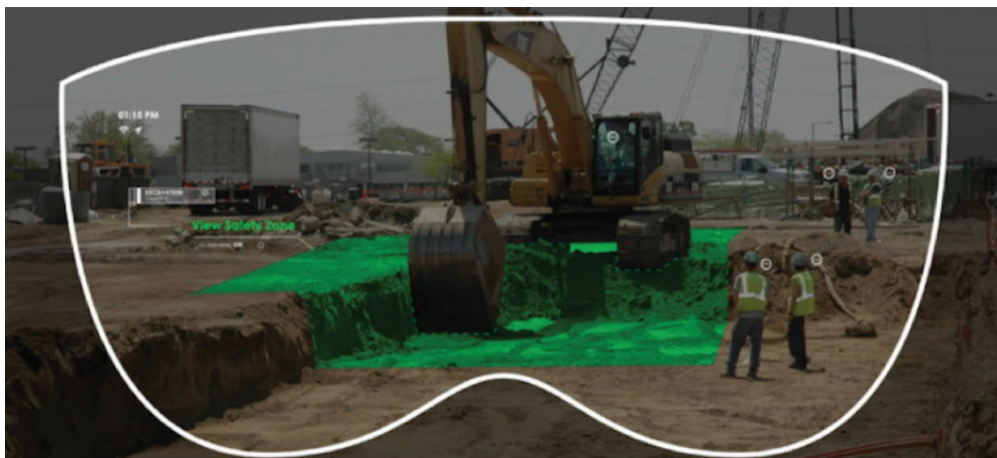
Fig. 24: Counting labours by AR-based wearable goggles for construction safety. Source: (International, 2017).
