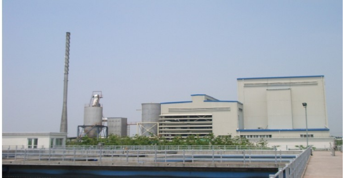
Figure 5: Shidongkou Municipal Wastewater Treatment Plant, 26 th of July 2011
