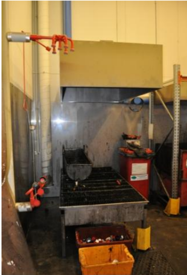
PICTURE 5: Ventilation system and shower
