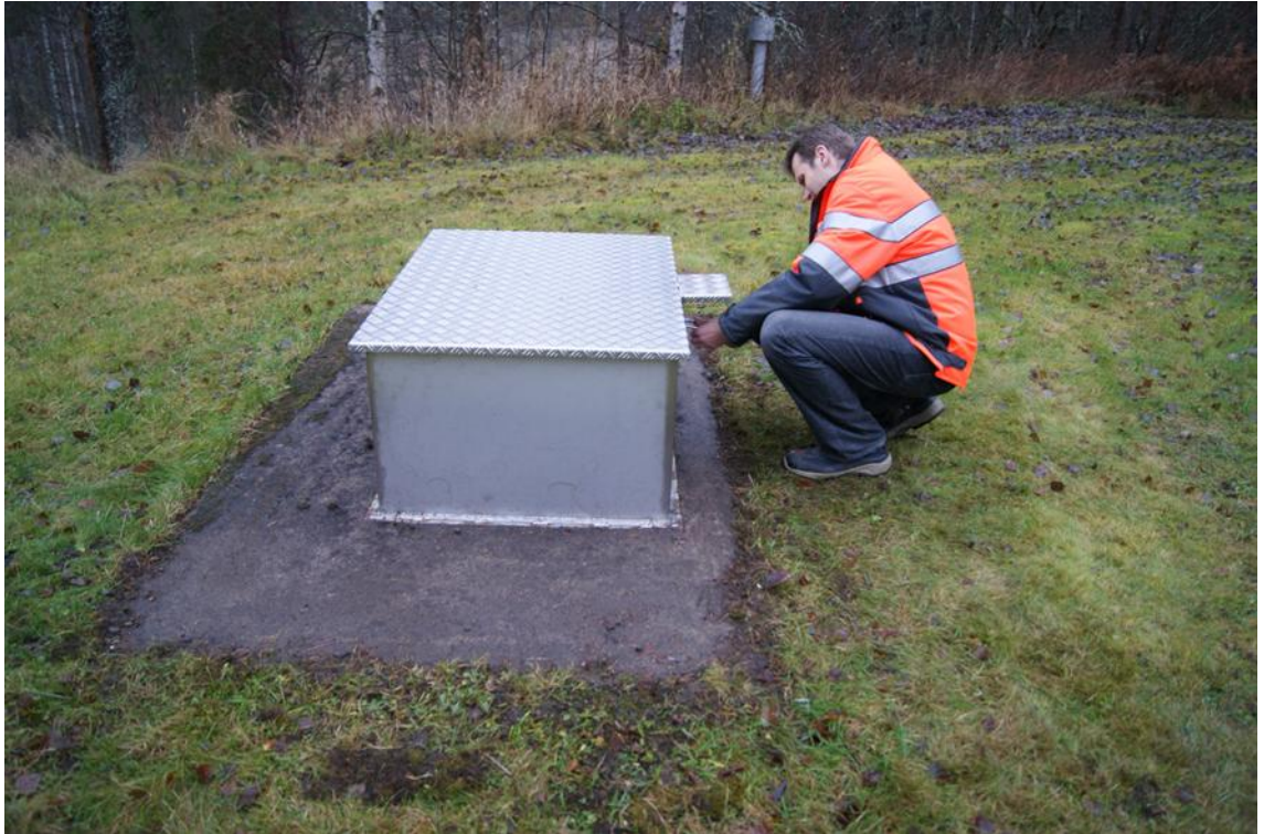
Figure 9. The area of clean water tanks (situated underground)
