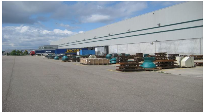
Picture 1 Tongeren warehouse
