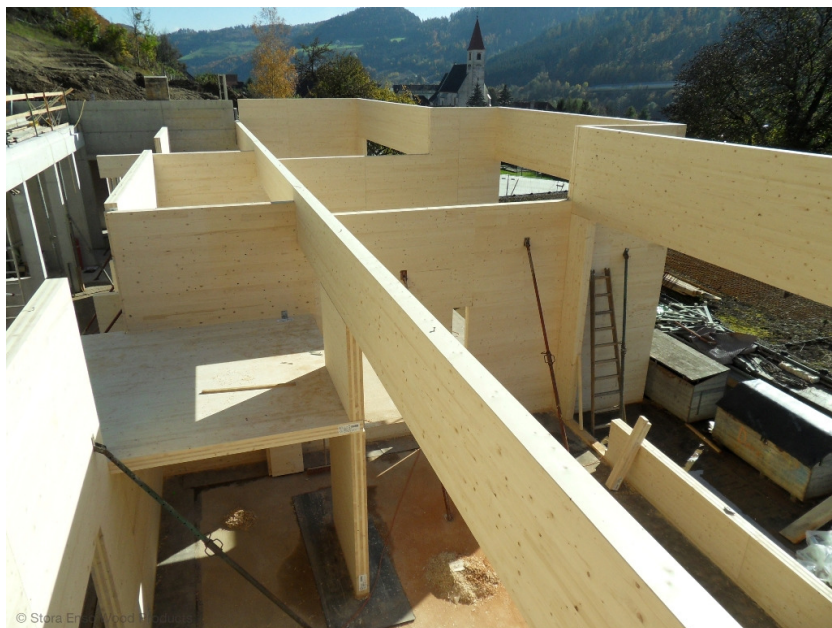
Figur 11 CLT byggande (Stora Enso – Public buildings, 2008)
