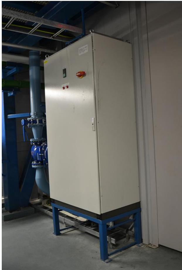
Figure 11. The control cabinet installed.
