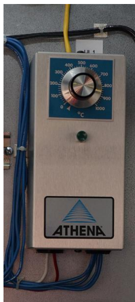
Figure 17. Athena controlling the high limit of the heater.
