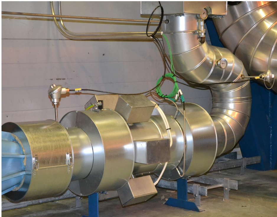
Figure 28. The electrical heater insulated and finished
