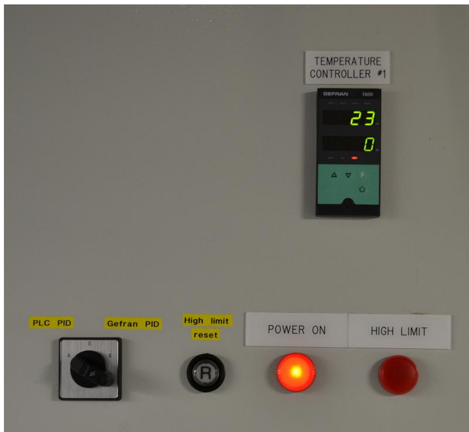
Figure 18. A PID regulator switch and a high limit reset have been added in the control cabinet's door.
