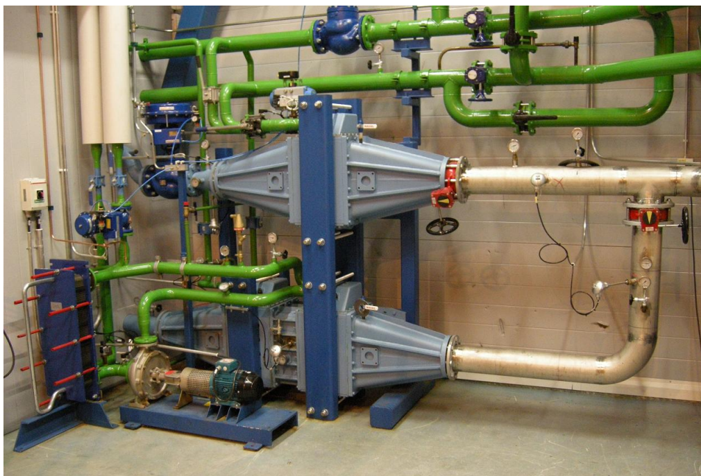
Figure 5. The charge air cooler and heaters in the test cell.
