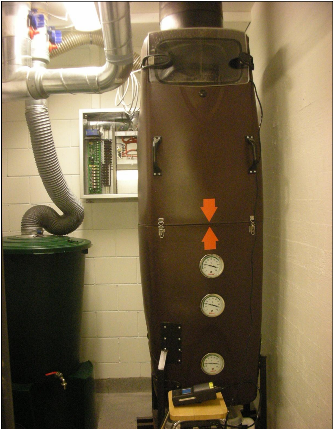
PICTURE 2. Dual-layer dry-toilet composter (Right) with Naturum urine tank (left) and gas control system (back) at the basement (Photo: Pui Ki Tsang 2012)
