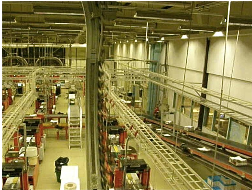
Figure 19 Alma Manu belt conveyor(loading)
