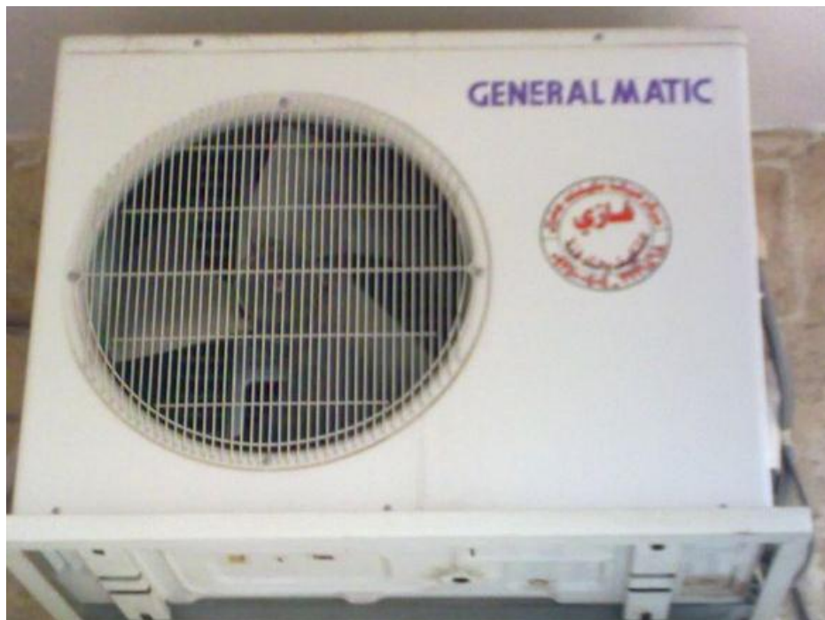
PICTURE 11. The outside part of the AC used in Aleppo for getting water.
