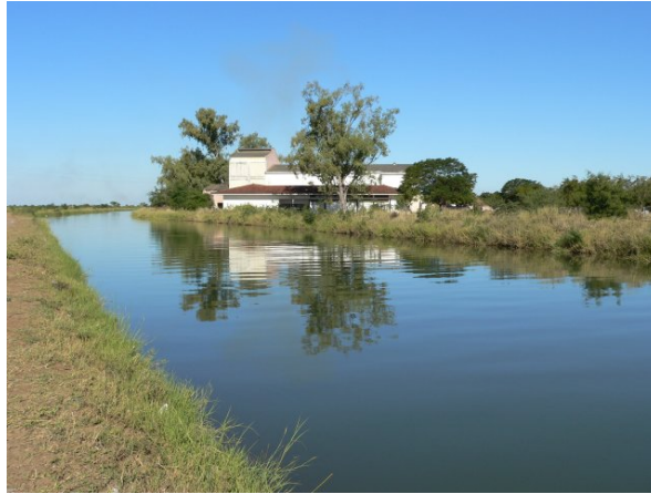
PICTURE 3. Main channel near the village of Chókwé (Source: Liisa Pekonen, 2007)
