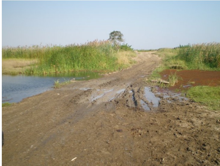
PICTURE 10. Ordinary road in irrigation system (Source: Anne Hakala, 2007)
