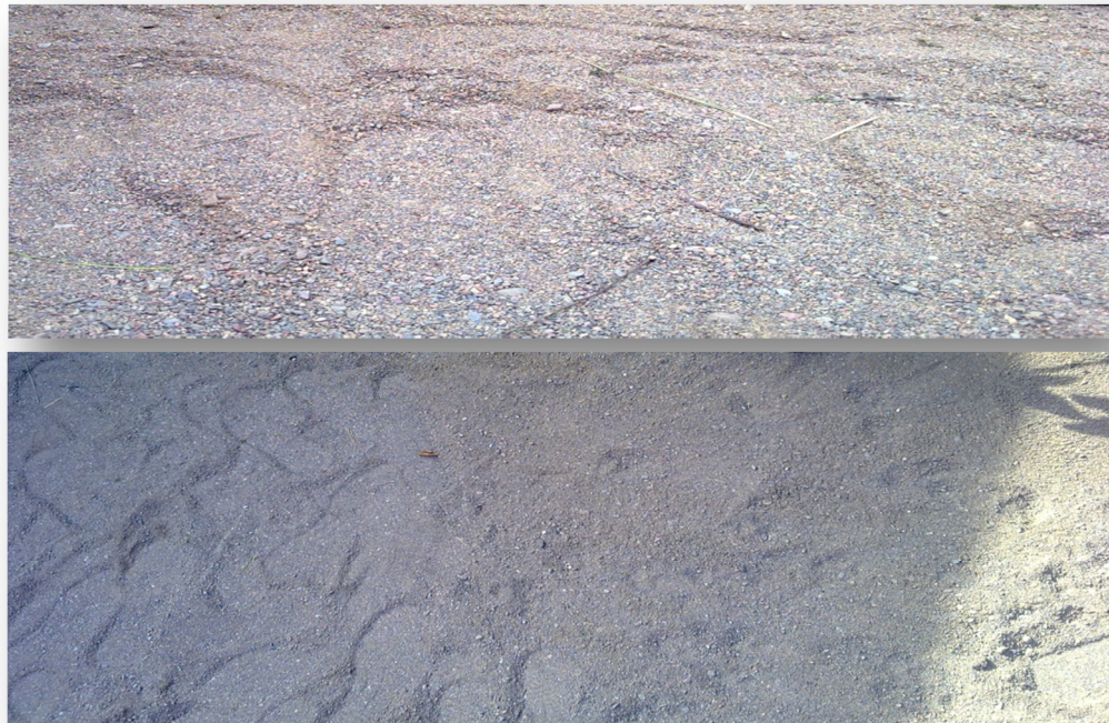
Figure 5: Bed sand before the installation of concrete paver
