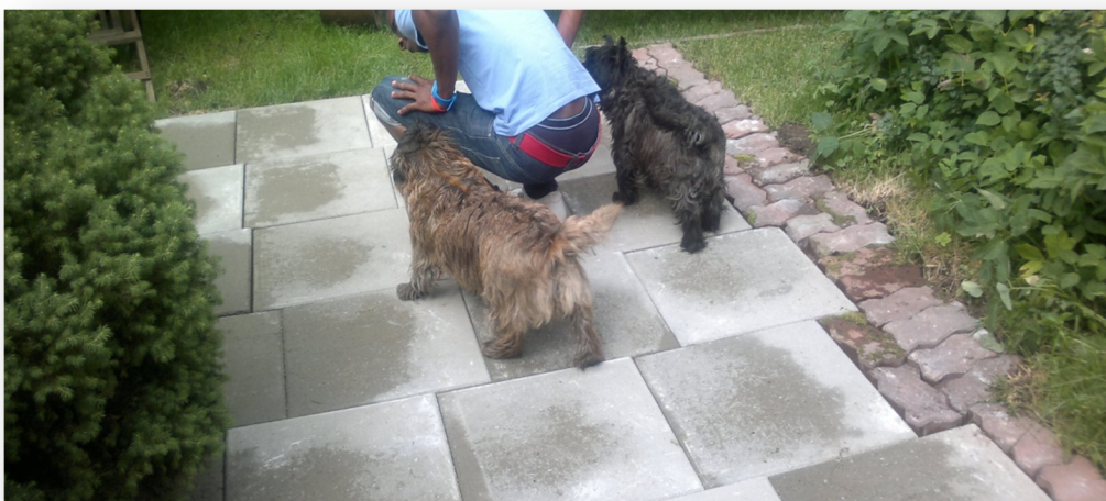
Figure 10: Final installation of the pavers without compaction
