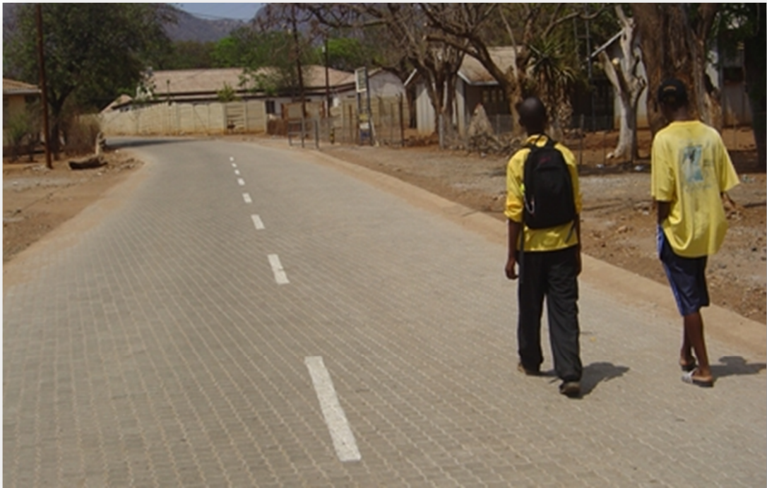
Figure 3: Modern rectangular interlocking concrete paving stones road in South Africa. [Tough Concrete Paver Meets Rural Road Challenge]
