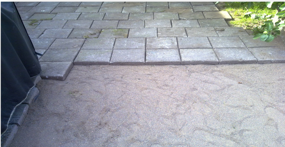
Figure 6: The front view during installation
