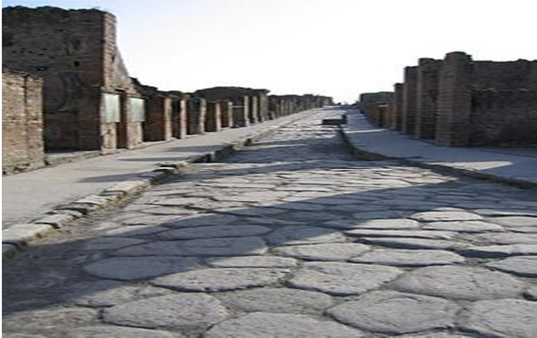
Figure 2: The rectangular Roman pave stones road in early 60's. [Roman Armies History Street in Pompeii]
