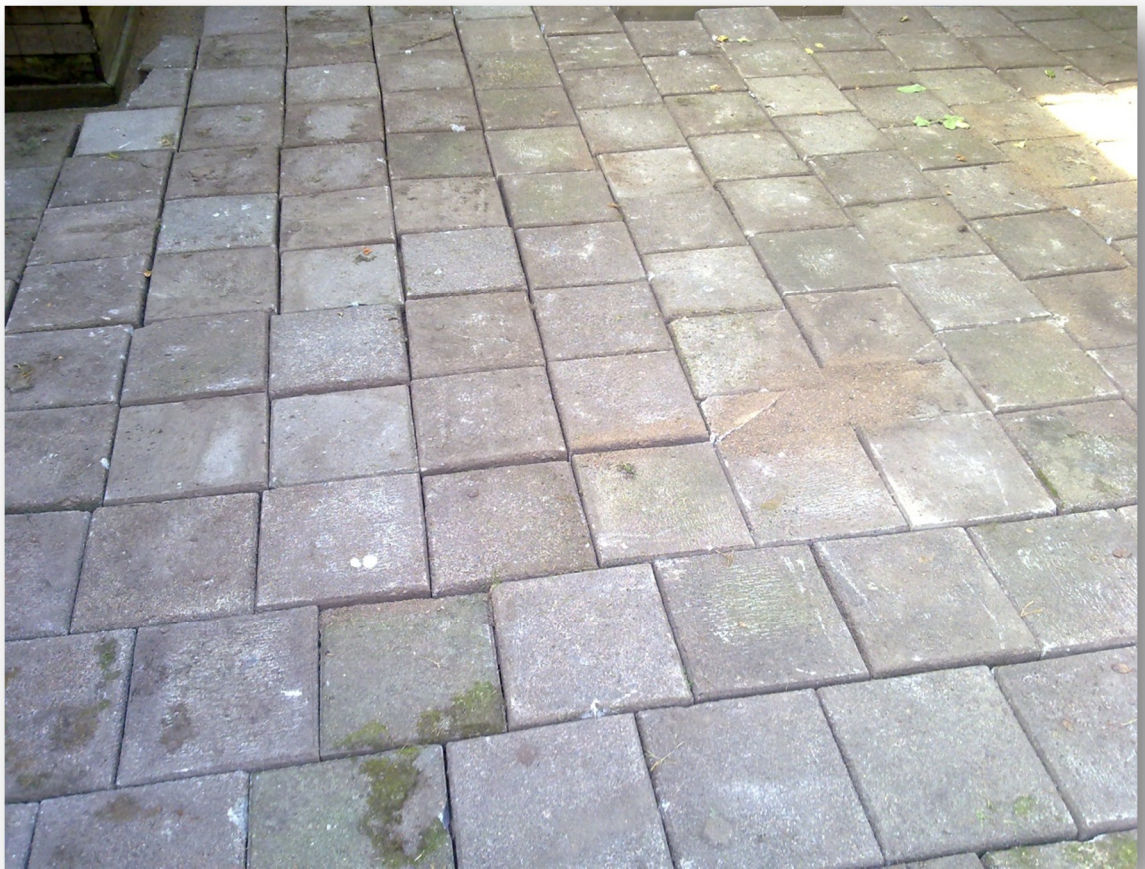
Figure 8: The plan view during the installation
