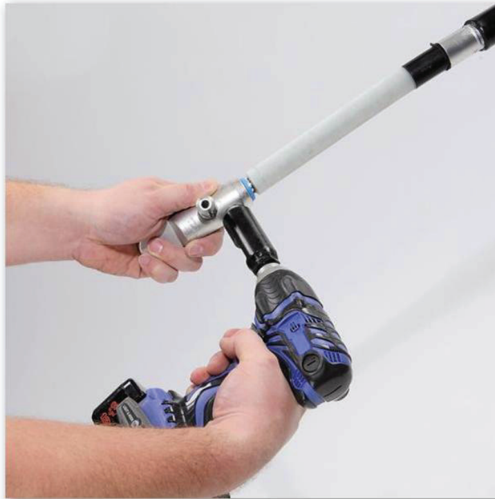
Picture 17. An example of installation of the cable lug using a photograph. [11]
