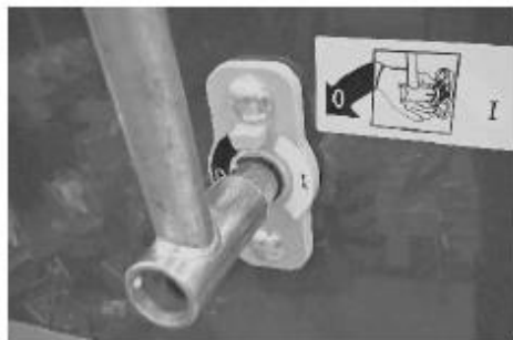
23 Put the operating handle on the splined end. Turn the handle anticlockwise to charge a mechanism opening spring (apply to A mechanism).
