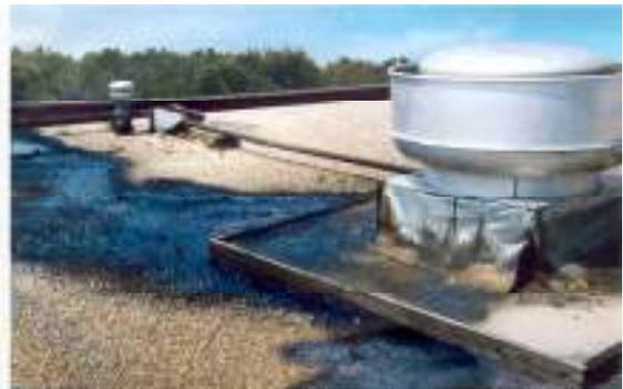
**Figure 5. Grease buildups on the roof flow on the building walls and pollute ambient and ground water /4/**
