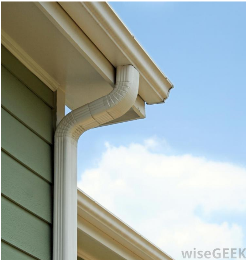
Figure 12. Water drainage systems (WiseGEEK 2021)
