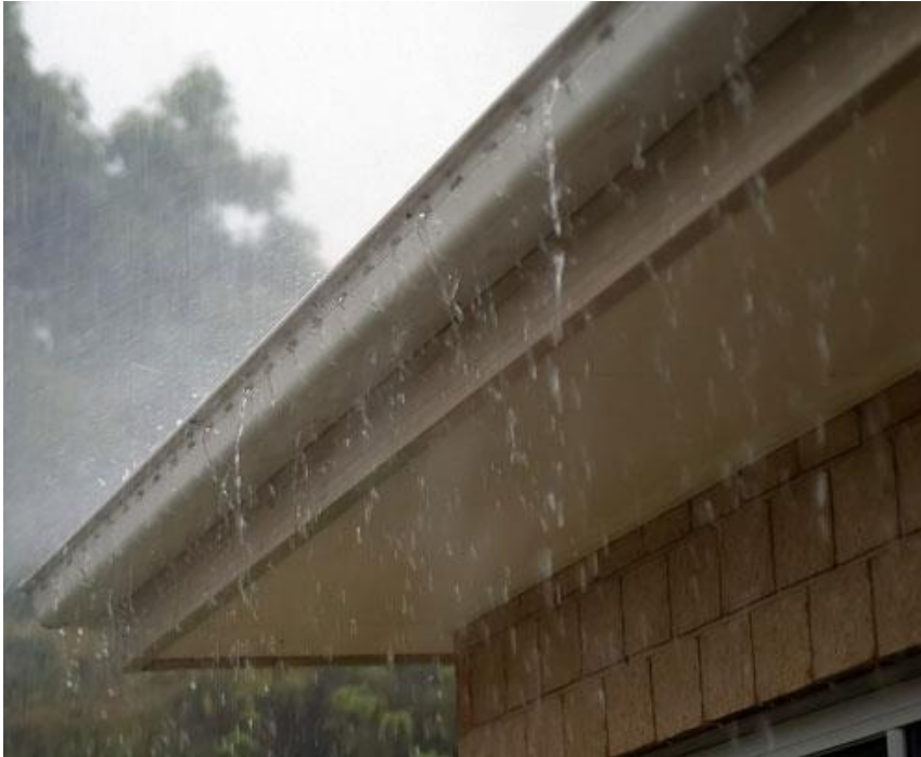
Figure 8. Eaves protecting facade from water (Tulsaprotech 2017)
