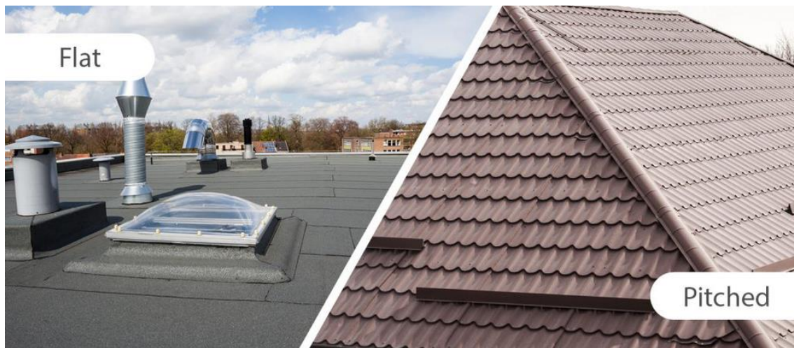
Figure 7. Pitched roofs versus flat roofs are safer choice in the face of moisture (A9architectur 2019)
