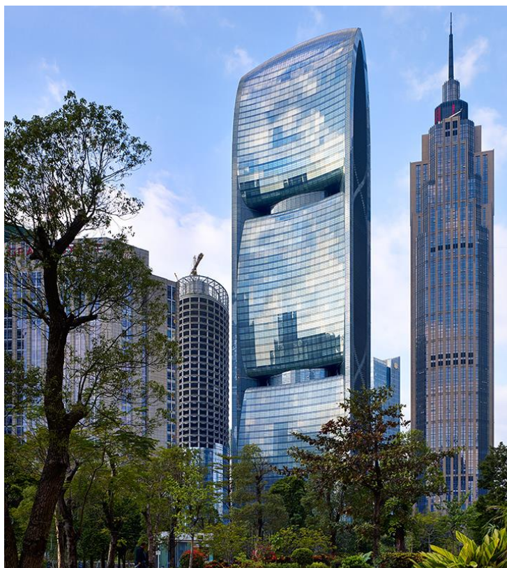
Figure 4 Pearl River tower (Placetech, 2021)
