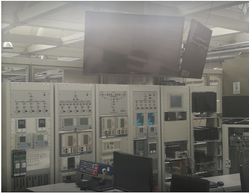
Figure 7. Part of Technobothnia.
