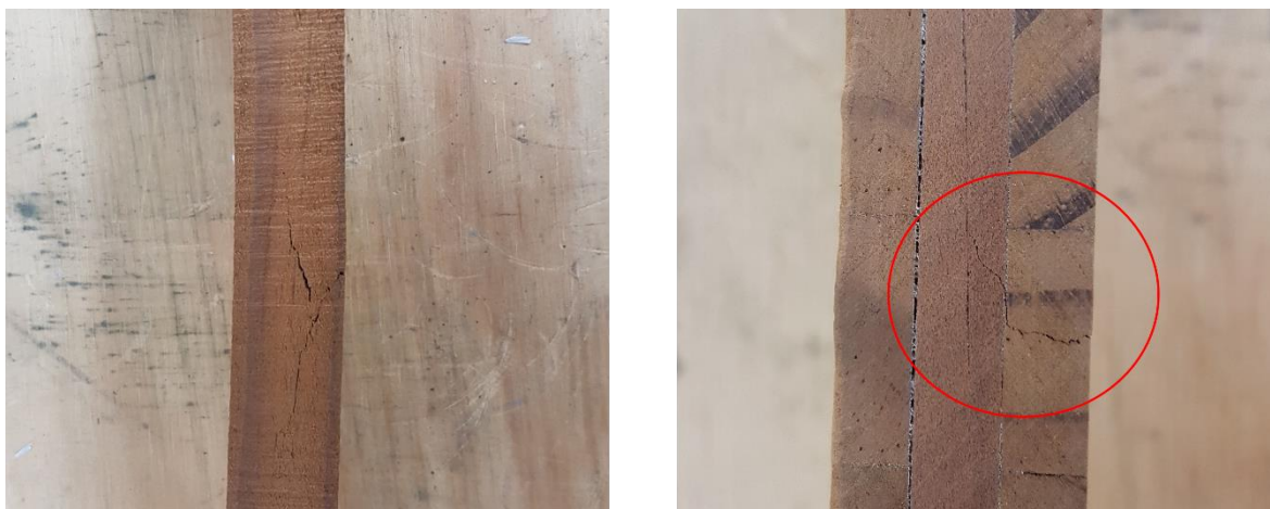
Figure 11. The failure after MOE/MOR test in mini-CLT and glulam (Lee, 2021b)
