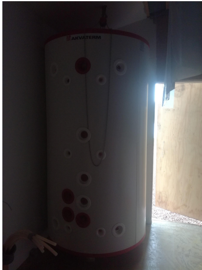
Figur 4. Ackumulatortank.
