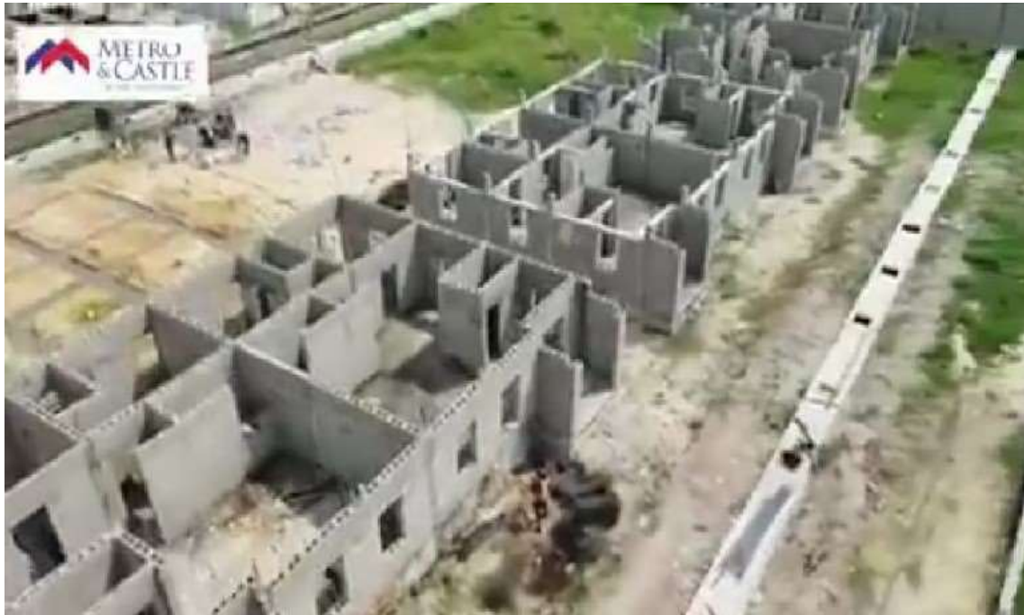
Figure 5. 2:Pictorial View of Work in Progress at the Site
