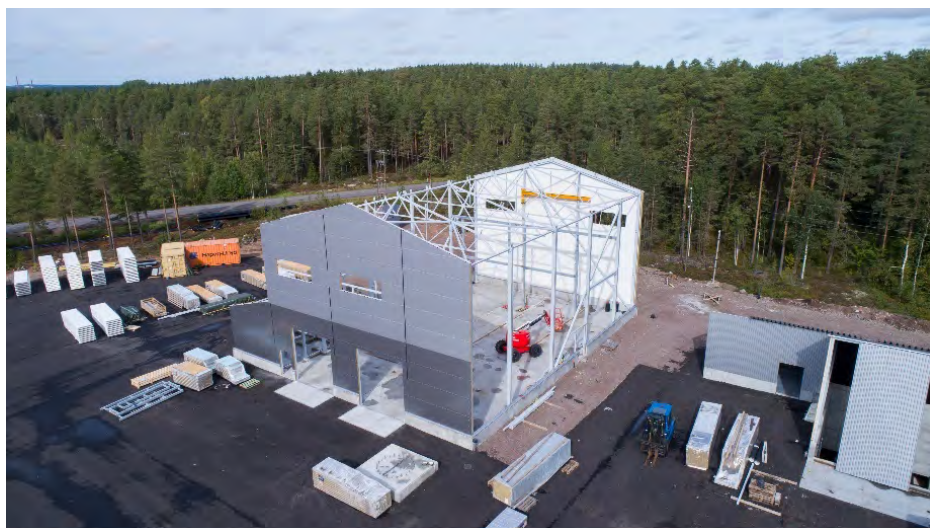
Picture 1. Wood chip thermal power plant under construction in autumn 2020. (Xamk)
