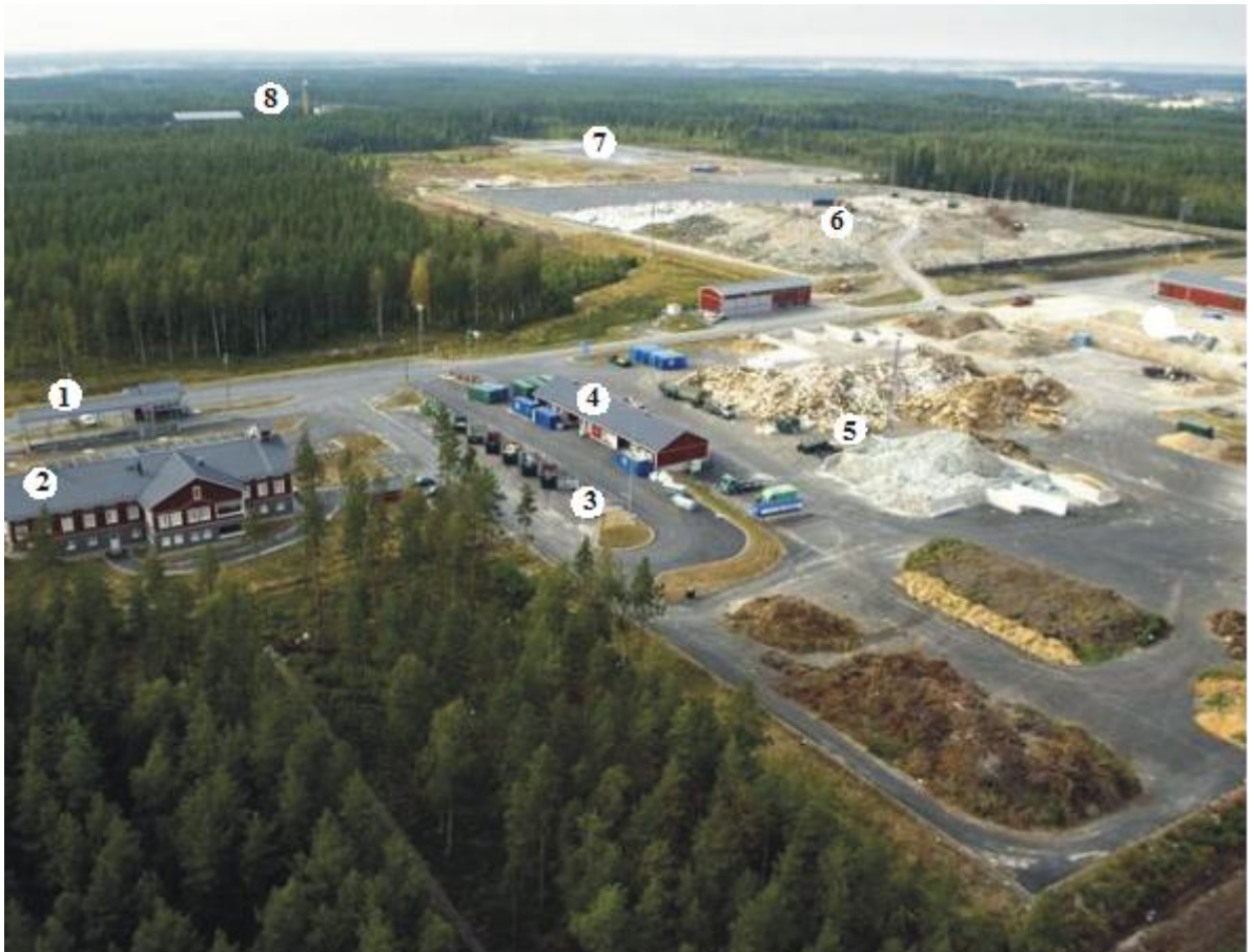
Figure 13: Waste Treatment Centre of Lakeuden Etappi
