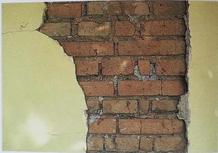
P-97 Painted smooth stucco over scratch coat, expanded metal lath, and brick
