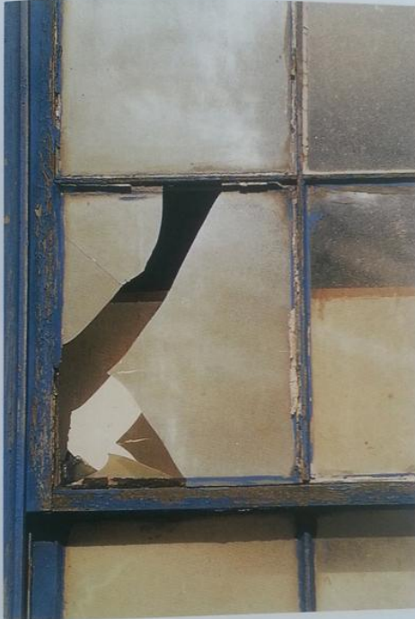
G-77 Broken window
