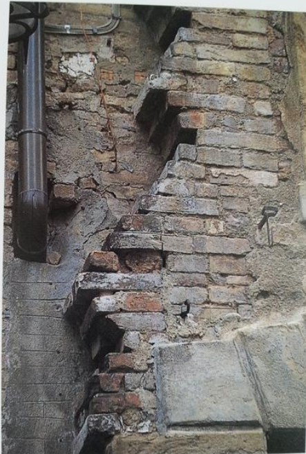
B-158 Roman wall, a portion demolished
