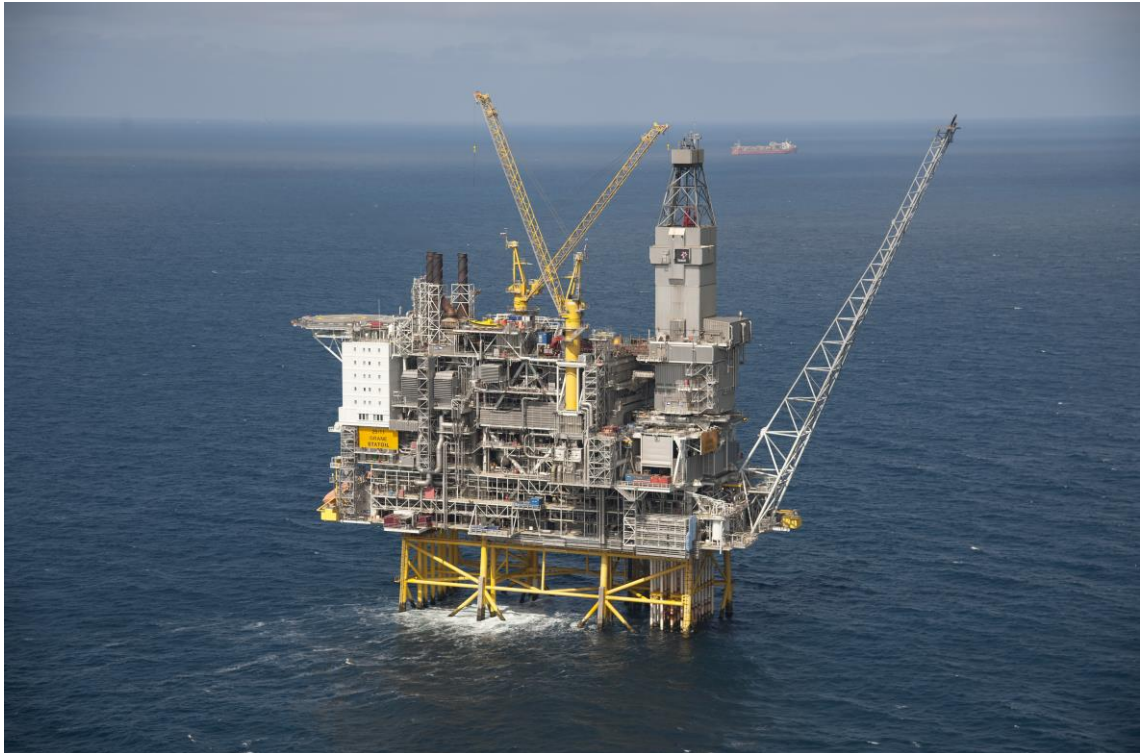
Figure 7. Grane platform. Photo: Øyvind Hagen/Statoil
