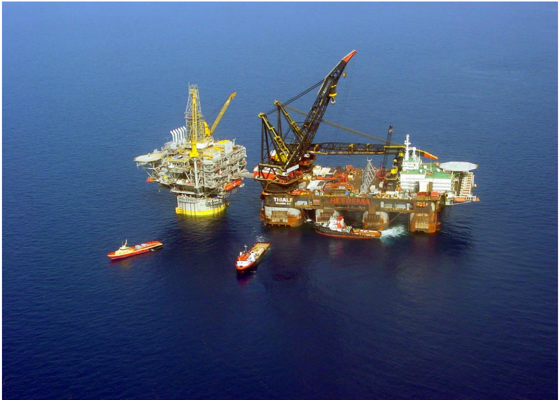
Figure 1. Deepwater construction vessel Thialf at construction site. Photo: Heerema
