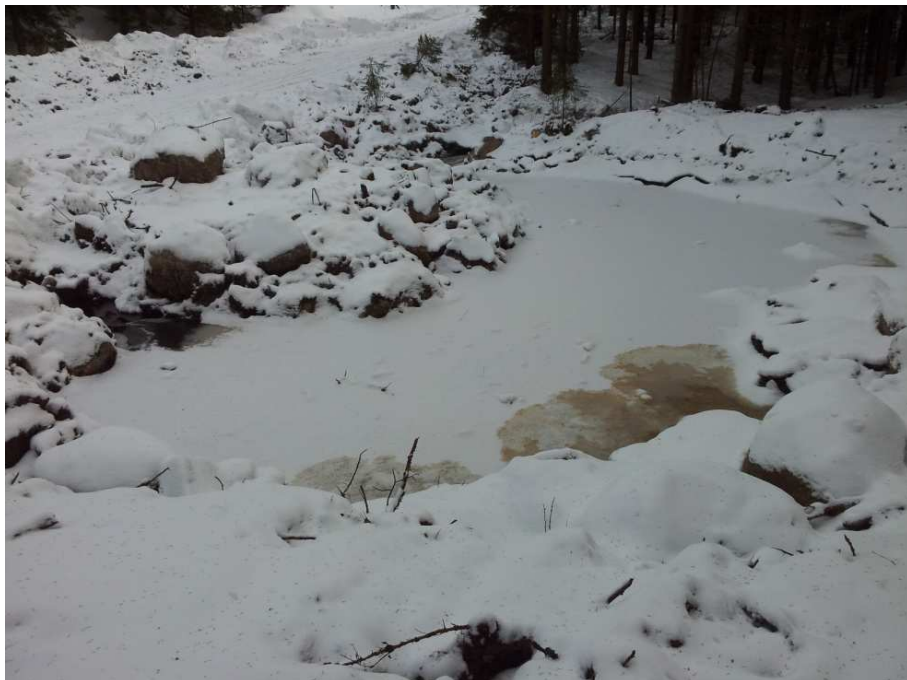
Figure 7 Sedimentation basin in point 1 of the plan. The inlet of the basin is located approximately in the middle of upper edge and the outlet in the middle left of the picture.
