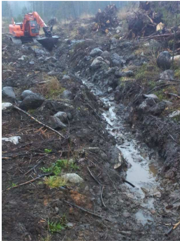
Figure 5 Excavation of the shallow drains below the Heinämäki hill.
