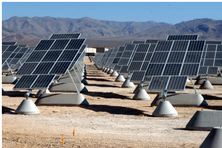
FIGURE 7. Panels tracking the sun in one axis (Nellis Solar power plant at NellisAirforcebase.USA)
