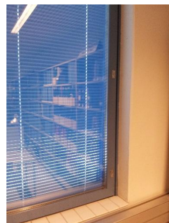
Picture 4. Single glazing window.
