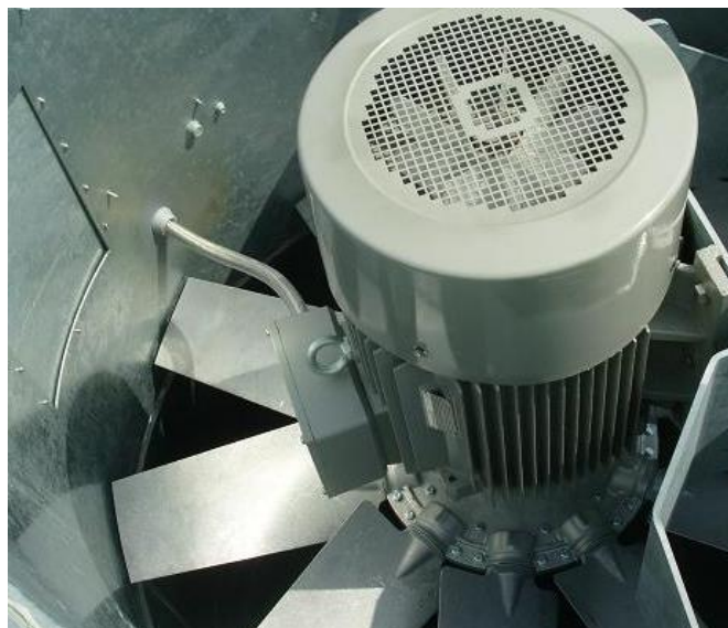
Figure 16. Fan motor with lifting lug.
