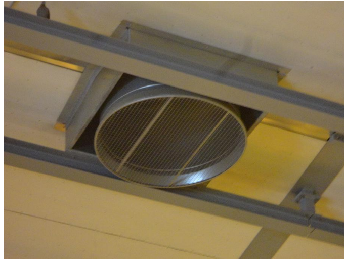
Figure 6. Roof ventilation unit's inlet cone and H-beams inside the engine hall.
