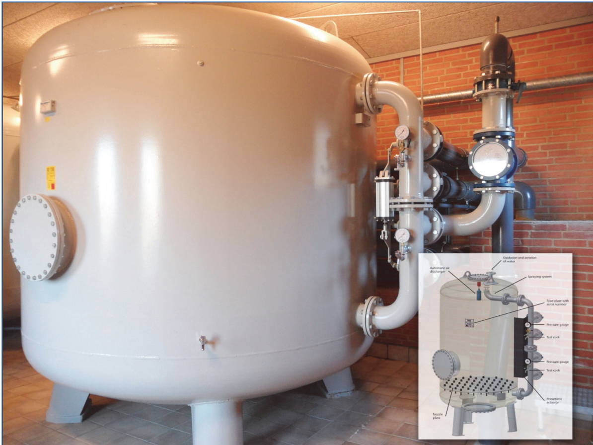
Figure 40 Multiple-media filters from the brand “Eurowater” at Pilegaardsvej waterworks. Scheme from Eurowater - description of pressure filter. Curtsey of Silhorko
