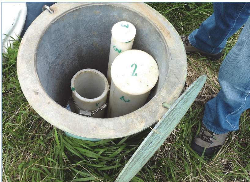
Figure 34 Observation well at Kolt-Hasselager area. Ewoud 17.05.2013
