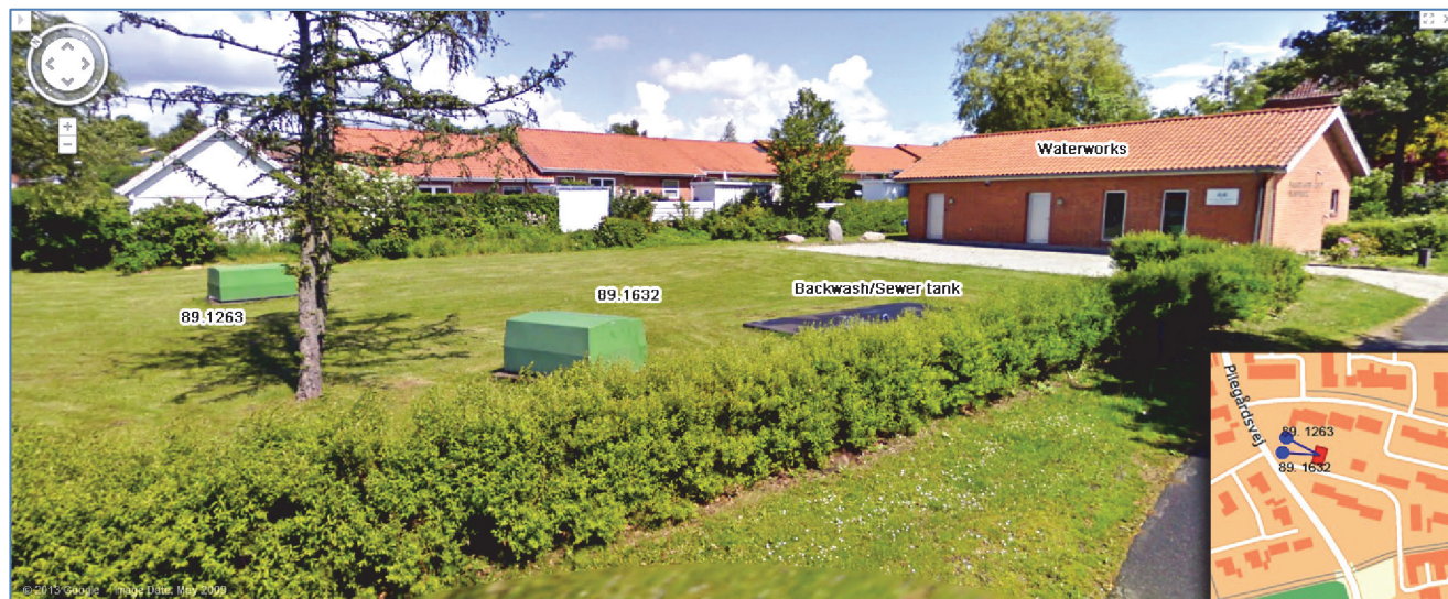
Figure 11 Pilegaardsvej waterworks exterior view. Base from the Street View, Google
