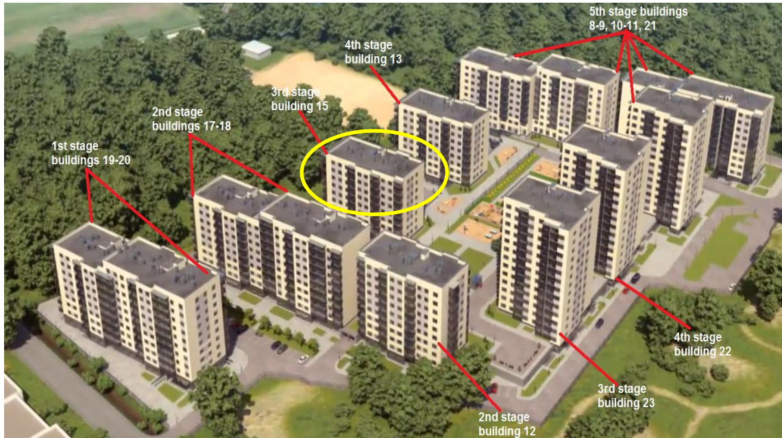
Figure 4.2 Building 15 in which the heat recuperation system was installed
