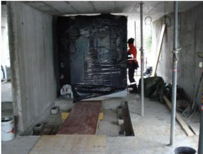
Figure 5.8 Settlement of the cabin to the final position.
