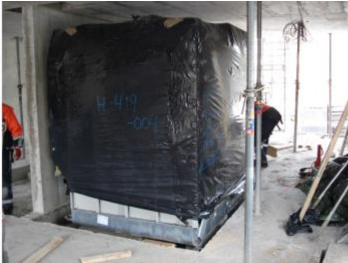
Figure 5.9 The view of the cabin after finishing of the mounting process.
