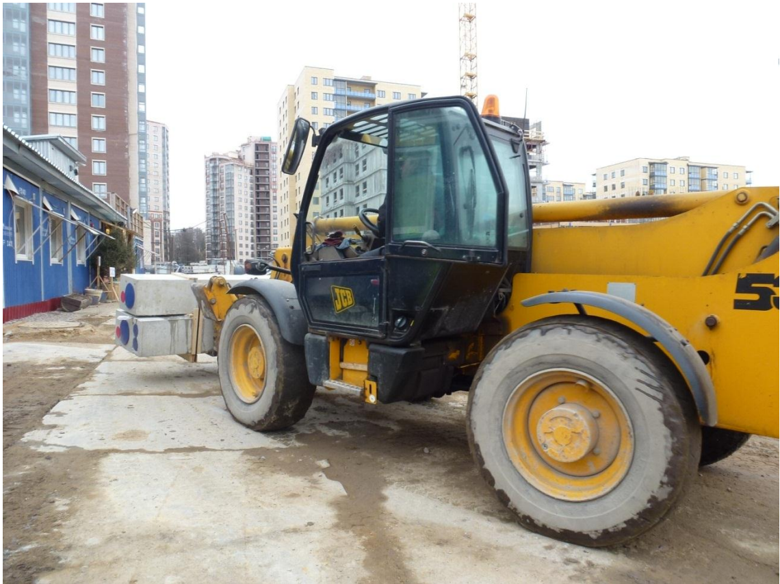
Figure 3.1 Transportation of Elpo to the construction site
