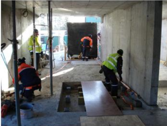
Figure 5.7 Moving of the cabing along floor structures and the final settlement.
