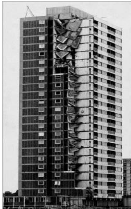
Figure 2.9. Ronan Point after collapse (failures.wikispaces.com)
