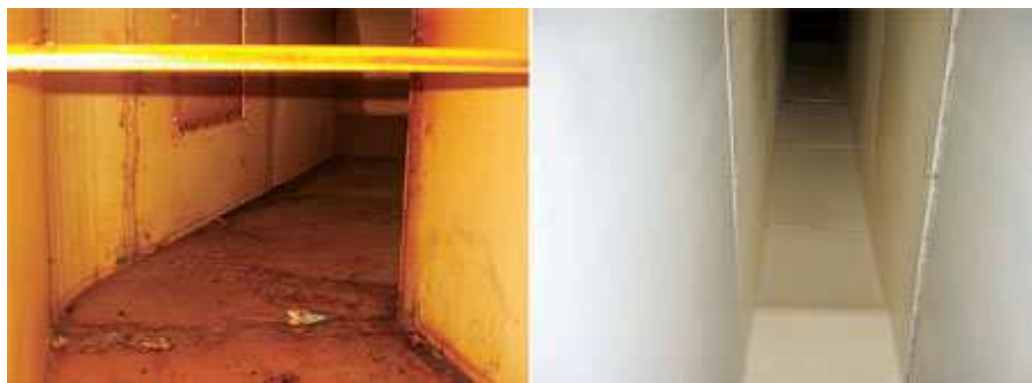
Figure 18 The result of using exhaust ducts without UV-technology (on the left) and with UV-technology (on the right) on a cruise ship “Queen Mary II” /8/
