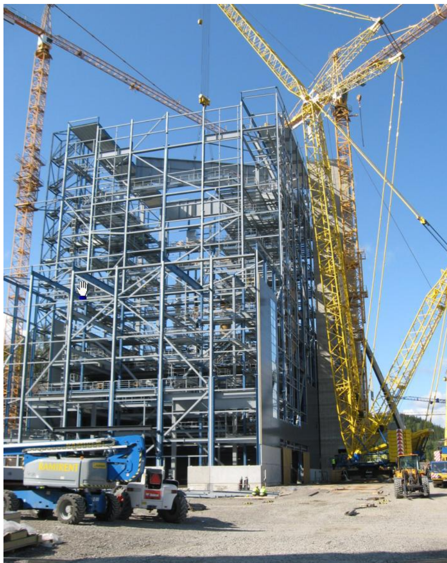
Figure 1: Boiler house steel frame and a simple outline bracing (Vänttinen 2012, 26.)
