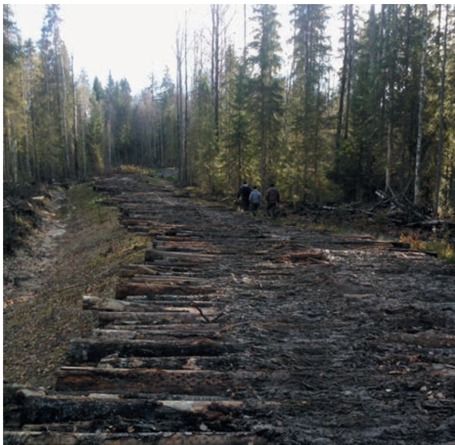
PICTURE 3. Forest road under construction in Podporoze (picture Kirsi Itkonen)
