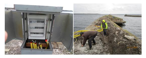
Pictures 35 and 36. The Sub-fuse box on quay and cable installations. © Leif Ortman
