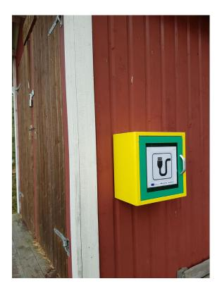
Picture 52. Northern pier: Box with sheltered USB-socket for charging mobile devices.  $\bigcirc$  Per-Olov Persson
