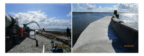
Pictures 47 and 48. ESB.2 Concrete casting ongoing and results for breakwater. © Leif Ortman
