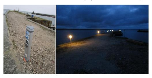
Pictures 37 and 38. New water, electricity and light service posts on the pier at Bläse Kalkbruk.  $\bigcirc$  Leif Ortman
