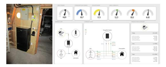
Pictures 32 and 33. Ferroamp inverter, main fuse for system and other gear installed and monitoring dashboard view. © Leif Ortman and Teemu Heikkinen (screenshot)
